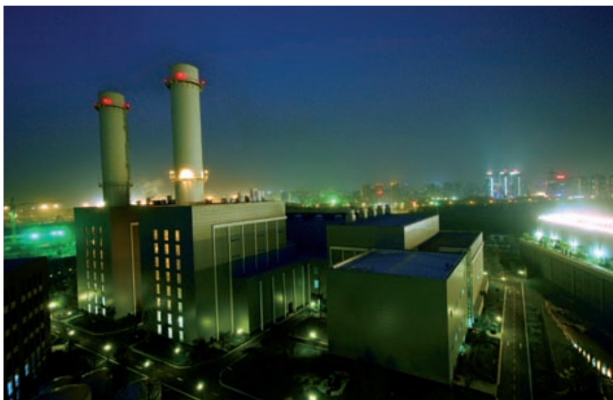
Energy efficient energy supply: the CDM project Taiyanggong CCGT Trigeneration plant in Beijing, China.
